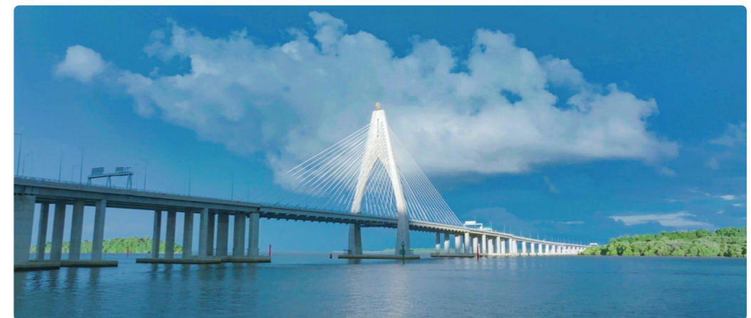
▲ Photo of the Temburong Bridge in Brunei
