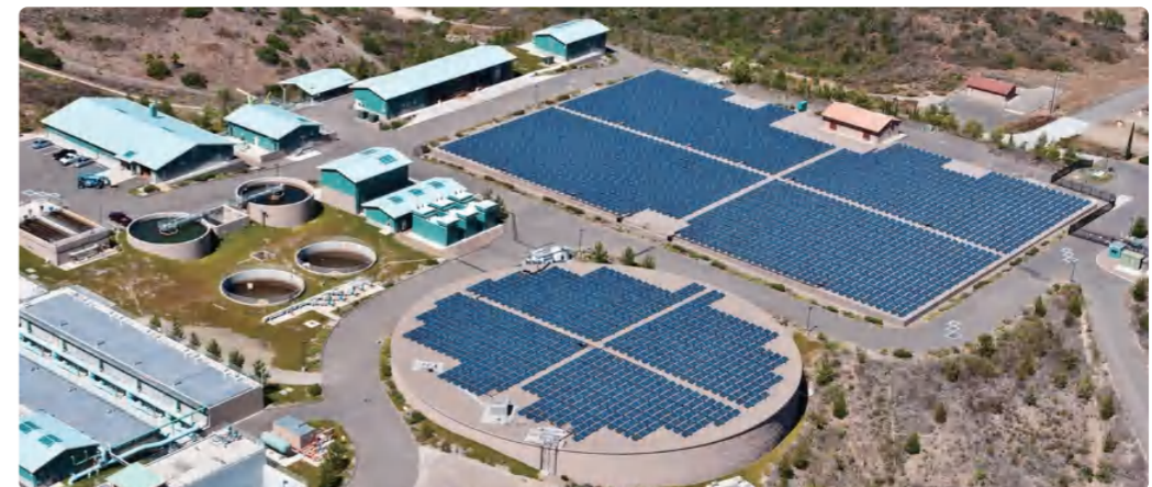
▲ Twin Oaks Valley Water Treatment Plant
