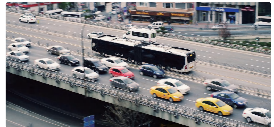
▲ Road conditions in Tartu, Estonia
