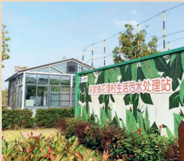
Sanitary sewage treatment station in Huapiao Village, East China's Zhejiang Province, October 29. Zhang Yuchai
