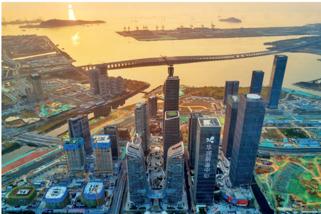
A view of the Qianhai Special Zone in Shenzhen, South China's Guangdong Province, January 31. VCG
