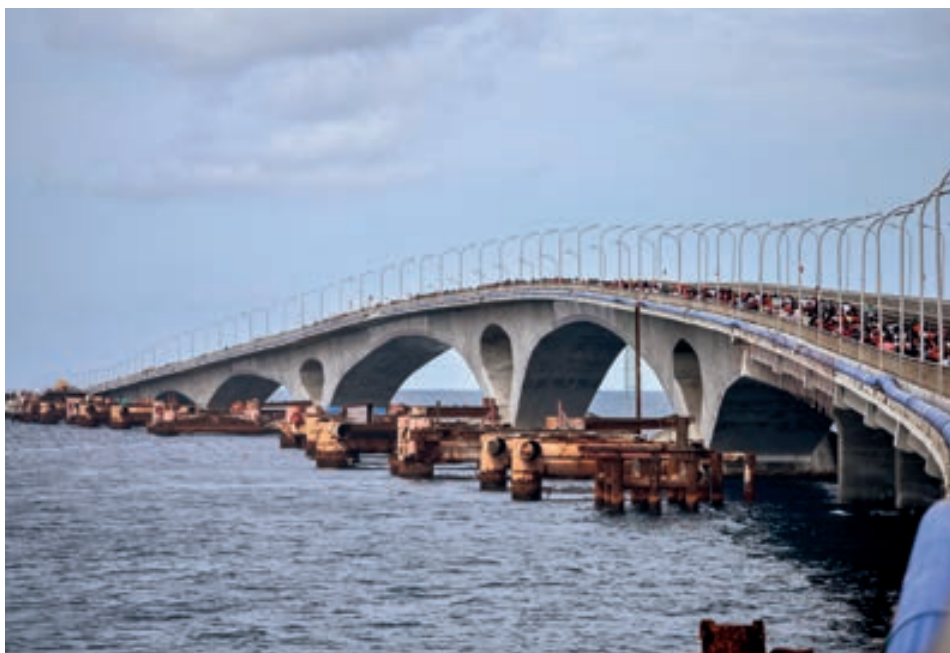
The newly opened China-Maldives Friendship Bridge is officially named "Sinamale Bridge" on September 18, 2018. VCG
