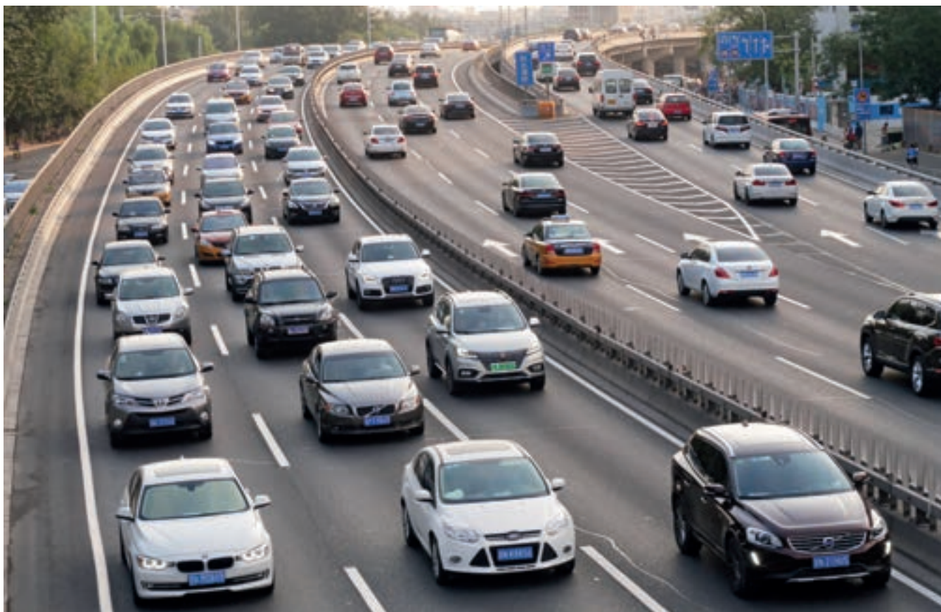
The vehicle stream on Jishuitan Overpass on the morning of September 25 in Beijing VCG
