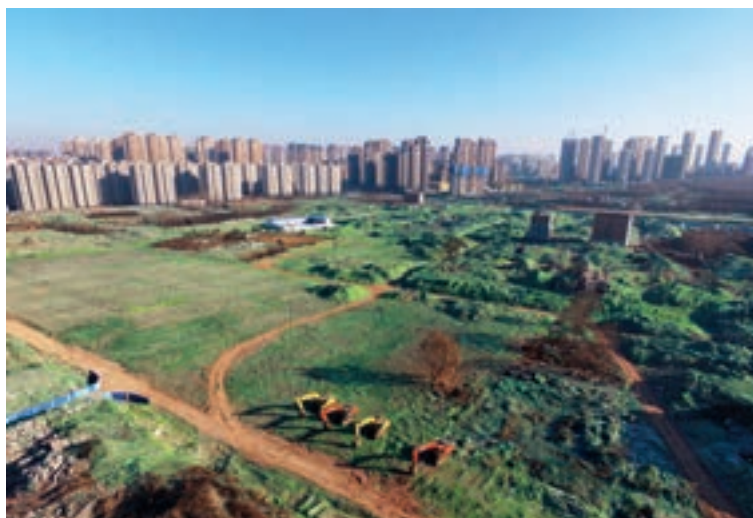
A demolition site is covered by nets to minimize spread of dust in Chang'an District of Xi'an, capital of Northwest China's Shaanxi Province, December 20, 2017. Shao Rui
