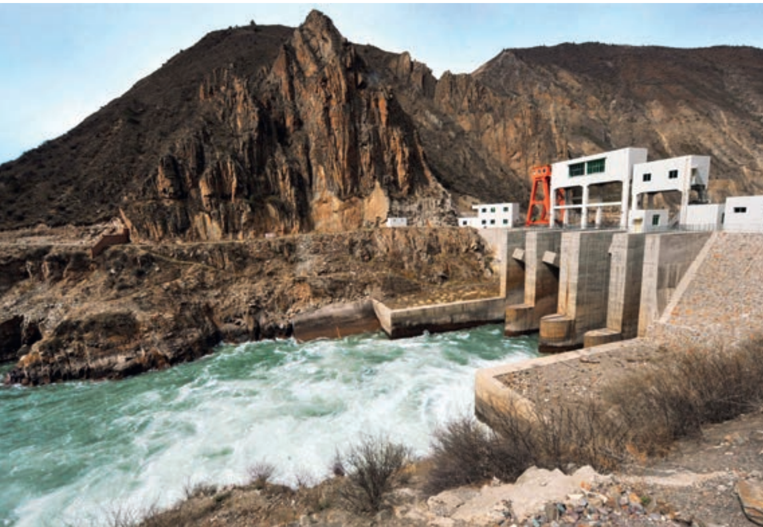
Qamdo Jinhe hydropower station, located along the upper reaches of Lancang River in Tibet Autonomous Region, is a key power construction and aid-for-Tibet project during the 10th Five-Year Plan period and its total installed capacity is 60,000 kw. Chen Haining
