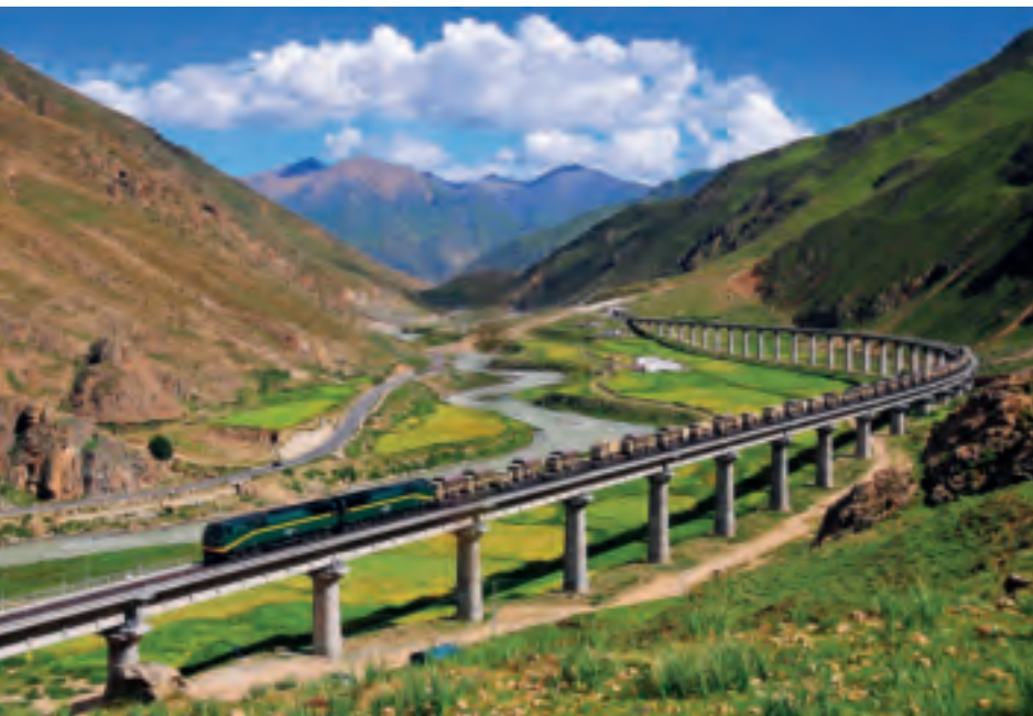
The 1,956-kilometer-long Qinghai-Tibet Railway, which connects Xining and Lhasa, is opened to traffic on July 1, 2006. The completion of the railway is regarded as one of the milestone projects in China's western development strategy. CFP
