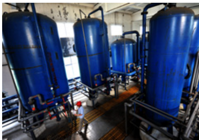
A worker passes a sewage water disposal system installed at a coal tar company in Fugu County, Shaanxi Province on May 16, 2012. The county pushes forward upgrading its traditional enterprises into a model of circular economy. Liu Xiao
