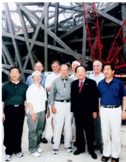
Mr. Stevens (3rd from the right), Daniel Ken Inouye (2nd from the left) and other US visitors pay a visit to the Bird's Nest – the National Stadium – which was still under construction. Zhong Sheng
