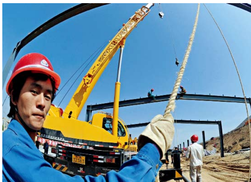
Employees of the China Railway 21st Bureau work at earthquake rescue and relief center at the Xining North Cargo Transportation Station in Qinghai Province on May 29. Hou Deqiang
