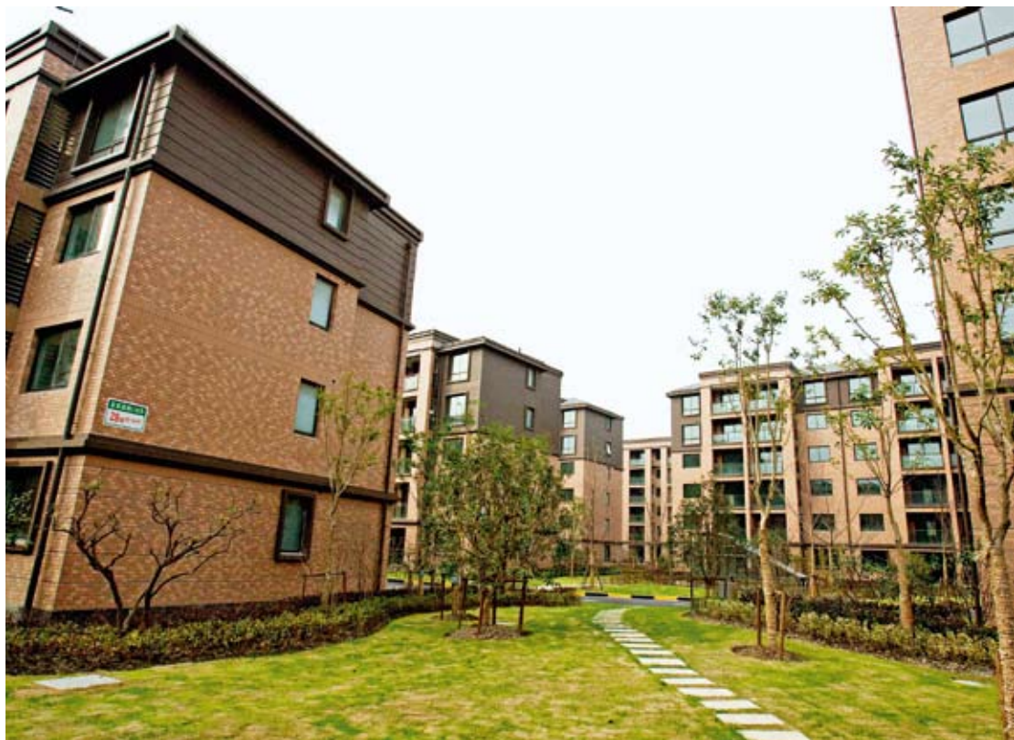
An indemnificatory housing project in Songjiang District, Shanghai. CFP
