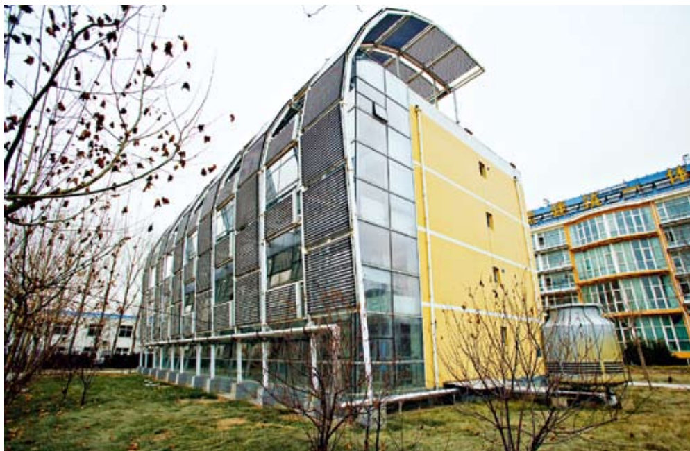
Solar energy equipment is installed on the top of buildings in Dezhou, Shandong Province. CFP
